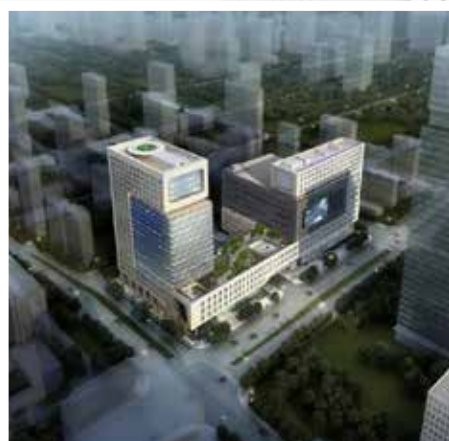
Shun Tong Building Ji'nan, China
